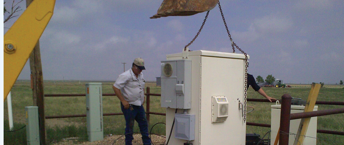
XIT's Construction Foreman, Rick Heiskell, supervises the setting of a cabinet, which houses electronics, during the Fiber-to-the-Premise construction in the Draper Community near Texline.
